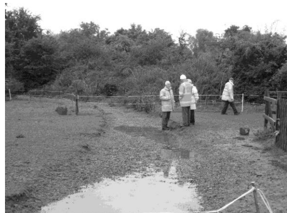
The puddles show that we still have drainage work to do: during Major Poyntz visit
