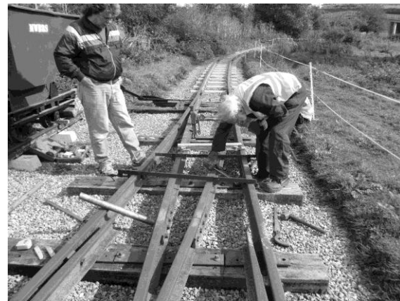
Pulling the point to gauge
