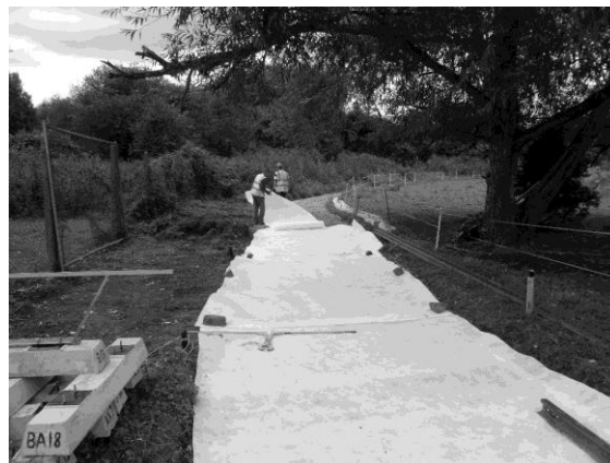
Laying Terram at the Station, 9 th August
