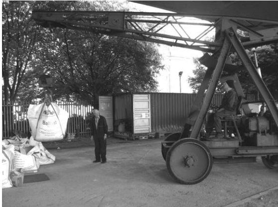
The first lift
