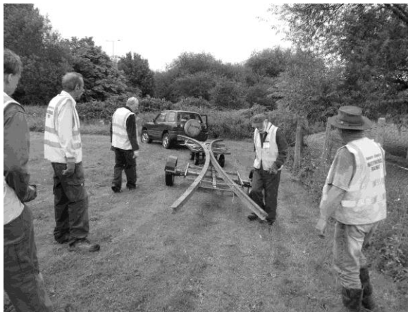
These were the tightest radius rails we have used and make quite a wide load
